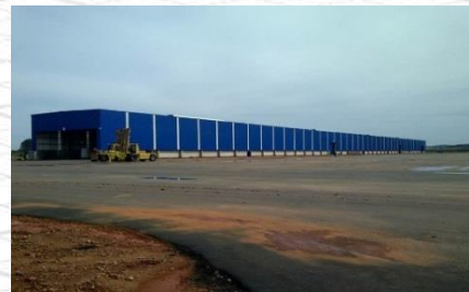
Steel Segment Guaíba - RS
