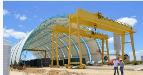
Concrete Tower Juazeiro - BA
